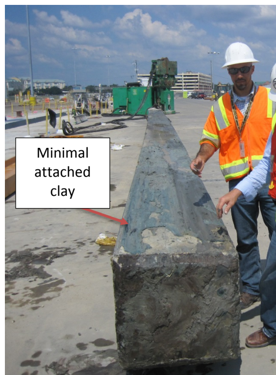
Photograph 1. Port of Gulfport Restoration Program - West Pier Wharf Upgrade (September 2013)
