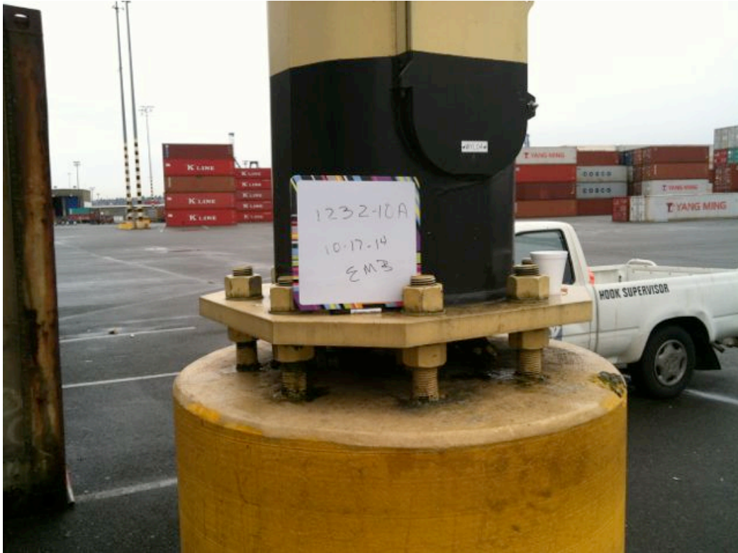
Photograph 11: Pier 4, Light Pole – Black/Yellow (Sample 1232-10P)
