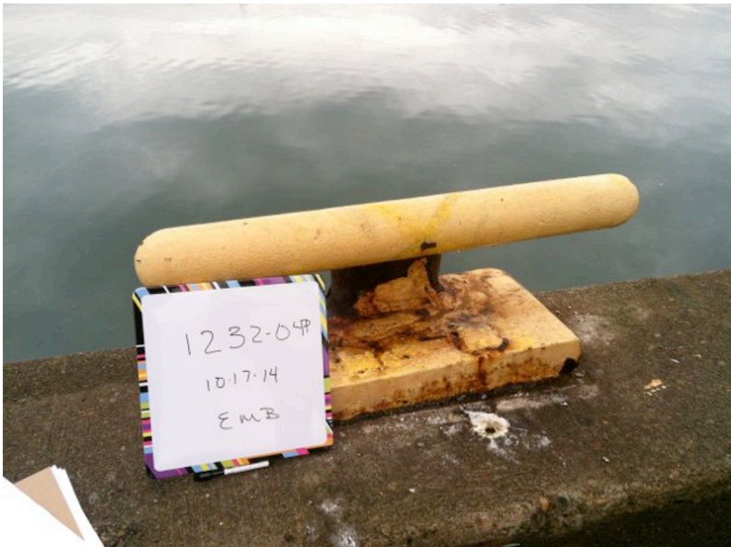
Photograph 6: Pier 4, Ship Cleat - Yellow (Sample 1232-04P)
