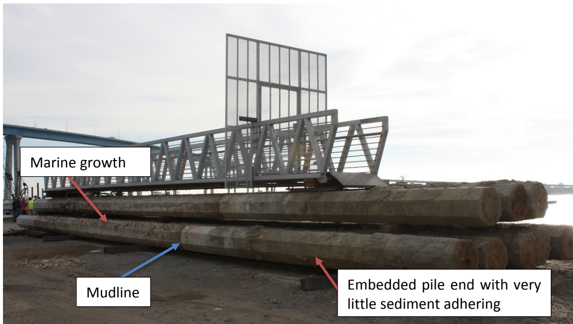
Photograph 2. Port of Long Beach Pier T Demolition
