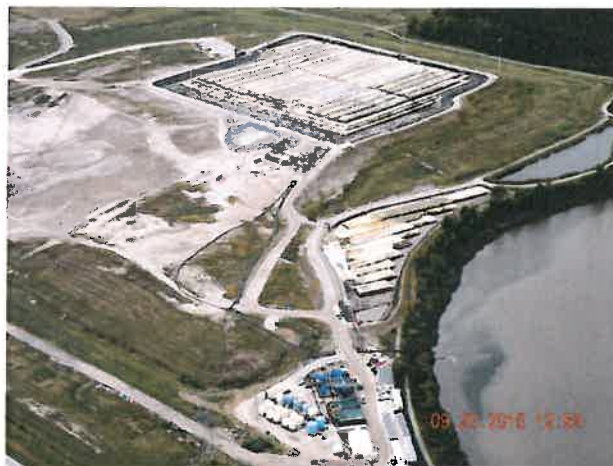
Figure 2. Aerial view of landside operations during active dewatering. The non-TSCA dewatering pad can be seen at the top of the photo, with the TSCA pad below and to the right, and the WTP pad at the bottom of the photo.
