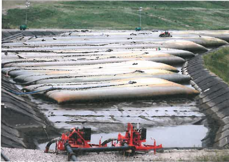
Figure 7. TSCA dewatering pad during active dewatering operations.
