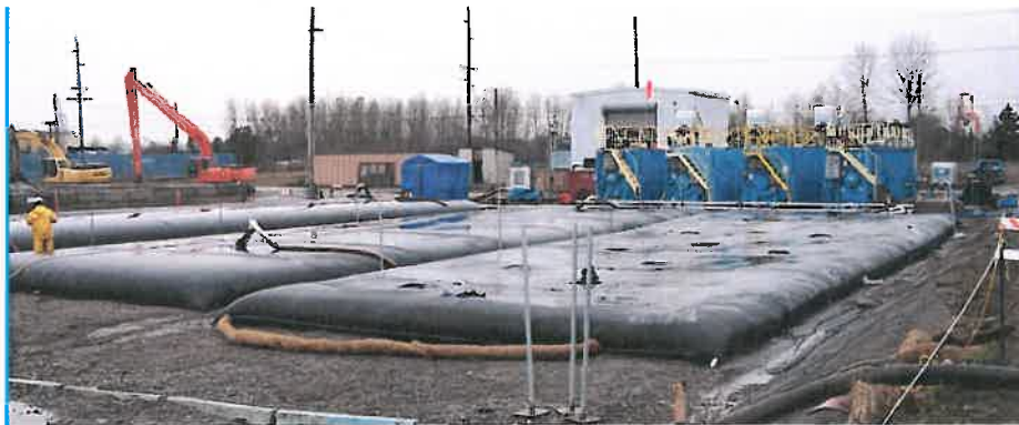
Figure 4. Geotubes with mixing tanks in background.
