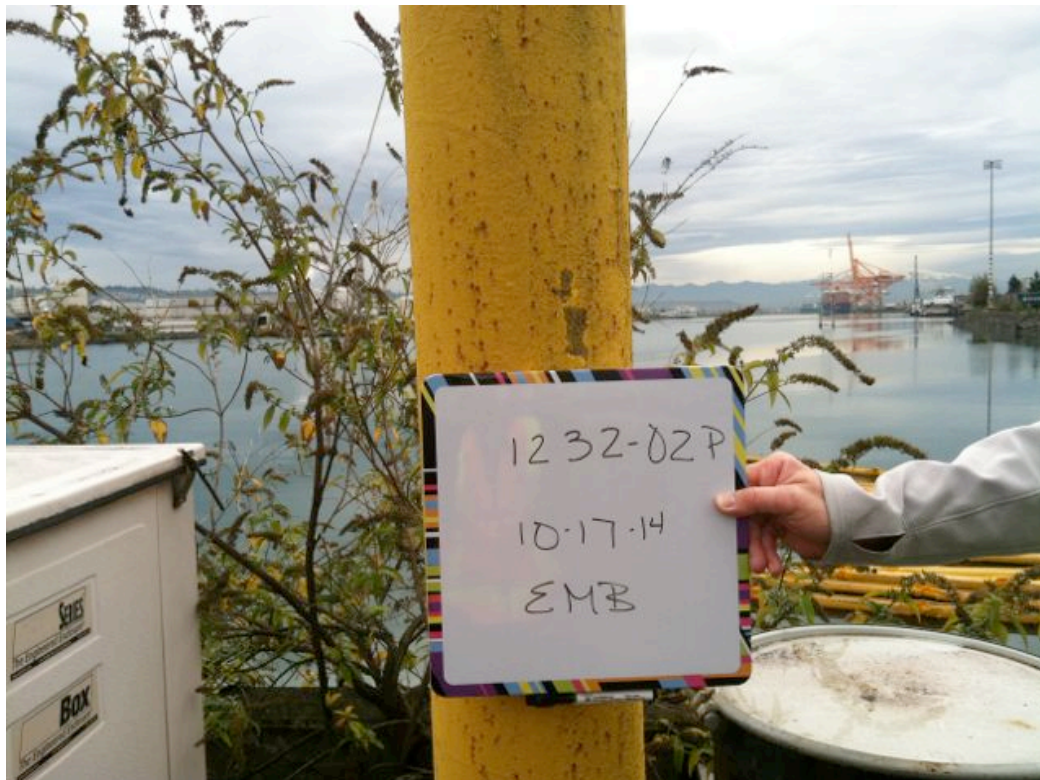
Photograph 4: Pier 4, Bollard Post - Yellow (Sample 1232-02P)
