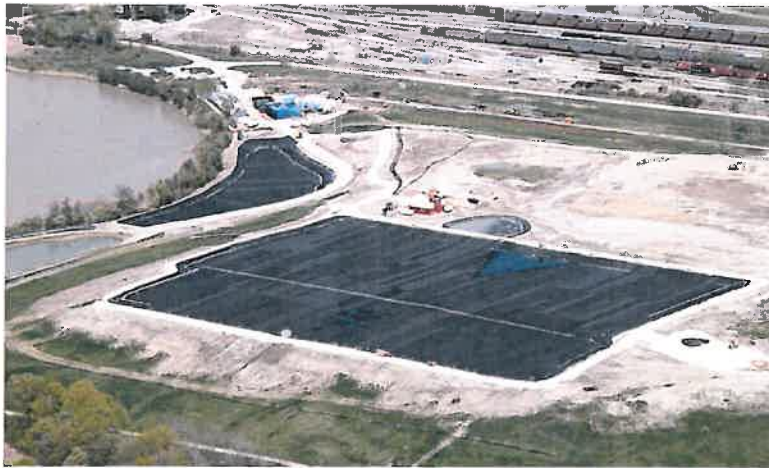
Figure 1. Aerial view of the site during construction of the sediment dewatering pads; the larger non-TSCA pad is in the foreground.
