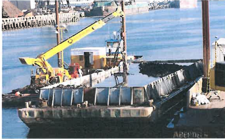
Figure 2. Barge dewatering system.
